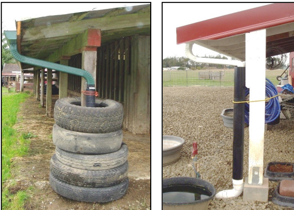
Old tires or thick plastic pipe can help protect downspouts from horse and livestock damage.
