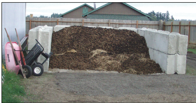
Waste storage structure for manure collection at a horse boarding facility
