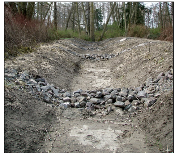
Typical infiltration ditch for aquifer recharge.
