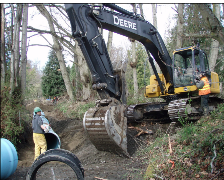
Irrigation pipeline installation.
