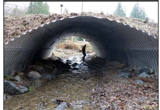
After: Culvert allows for unimpeded fish passage.
