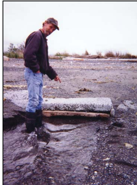
Figure 29 -Cassalery Creek culvert outlet (2000)
