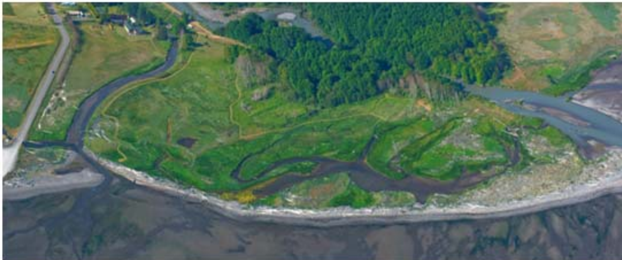
Figure 18 - Meadowbrook Creek outlet, slough, estuary, and Dungeness River (DOE photos, 2006)
