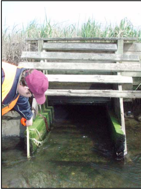
Figure 28 -Cassalery Creek culvert inlet (2007)
