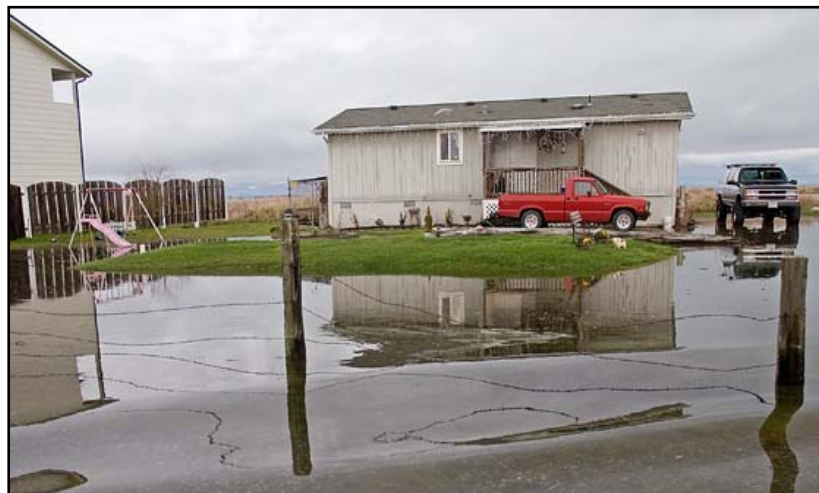
Figure 15 - Flooded septic drainfield along Three Crabs Road.
