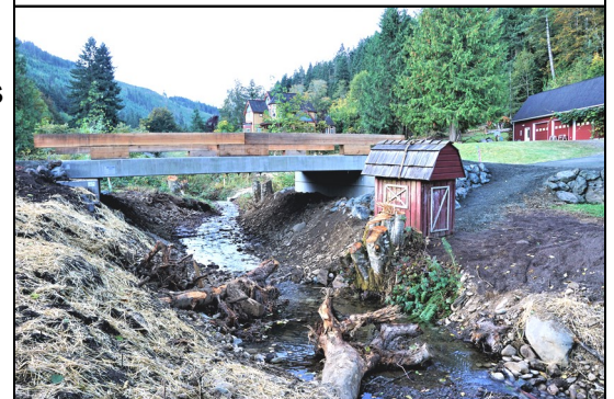
An undersized culvert (top photo) blocking fish movement on Tumwater Creek, was replaced with a bridge to allow for year-round fish passage. Family Forest Fish Passage Program (FFFPP) funds were utilized for the project.
