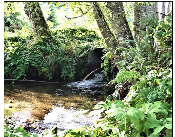
An undersized culvert (top photo) blocking fish movement on Tumwater Creek, was replaced with a bridge to allow for year-round fish passage. Family Forest Fish Passage Program (FFFPP) funds were utilized for the project.
