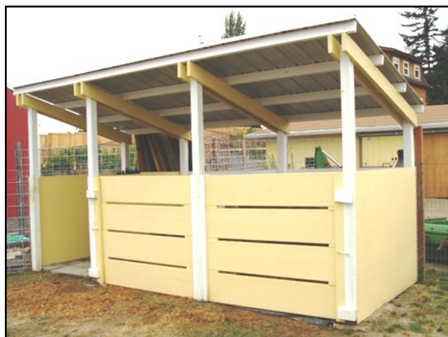
Wooden, 2-bin system with an equipment storage area on the far left, creates a tidy area to store manure, carts and manure forks.
