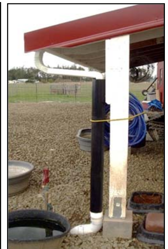
One farmer used old tires to protect fragile downspouts, another used a thick plastic pipe.
