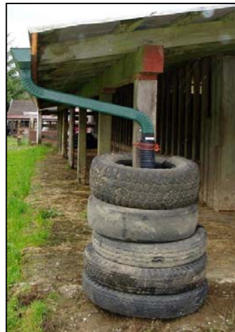
One farmer used old tires to protect fragile downspouts, another used a thick plastic pipe.
