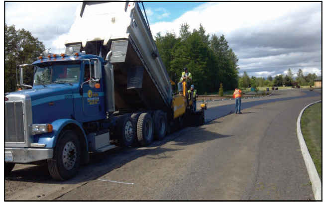
Lakeside Industries installing porous asphalt.
